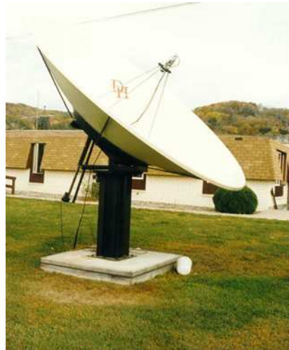
4.2 M Diameter Antenna with Single axes Gibraltar Mount
